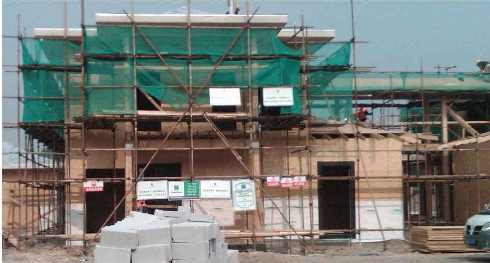
House framed with SPF lumber
