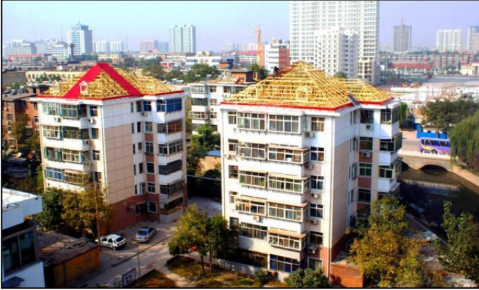
Wood truss re-roofing (east and north China)
