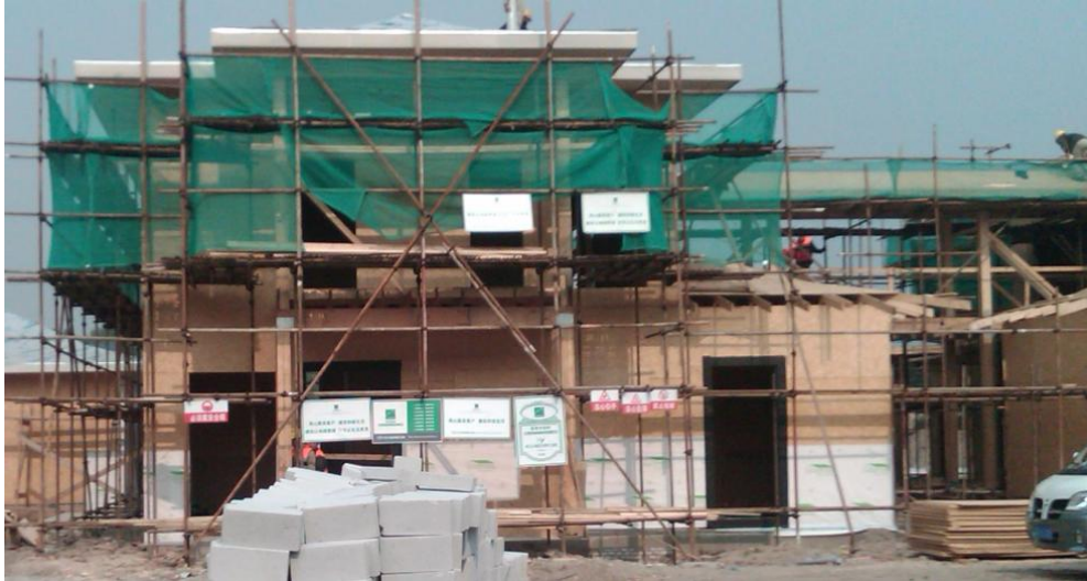
House framed with SPF lumber
