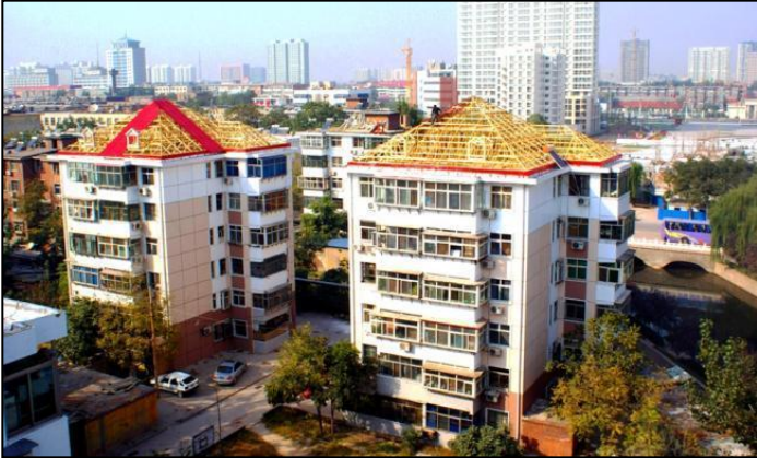
Wood truss re-roofing (east and north China)
