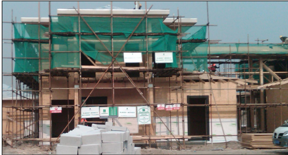
House framed with SPF lumber
