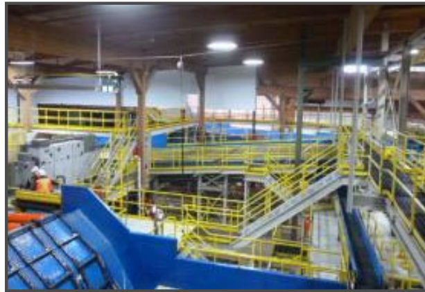
GRAND FORKS MILL REBUILD 2012
