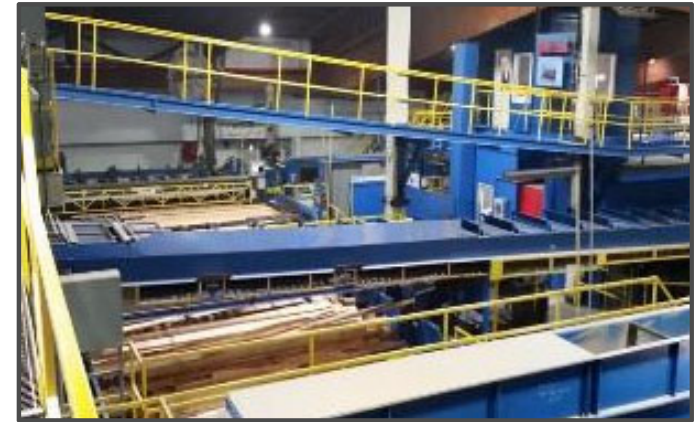
CASTLEGAR MILL REBUILD 2015
