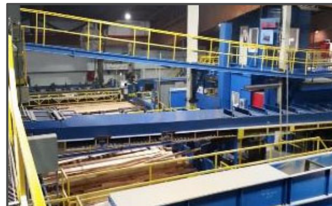
CASTLEGAR MILL REBUILD 2015
