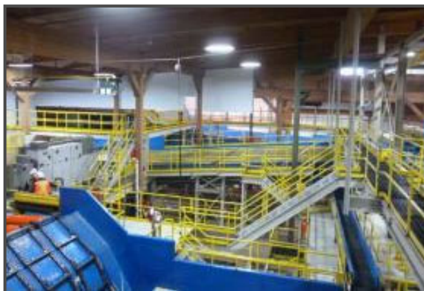
GRAND FORKS MILL REBUILD 2012
