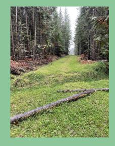
This deactivated road at the Adams Lake Lumber operation demonstrates noteworthy practices. Water management is evident in ditching and cross-drains. Grass seeding stabilizes soils and prevents ingress of invasive species and prevents the movement of sediment into water courses. Woody debris has been scattered onto the road surface as further water management and to provide wildlife habitat.
