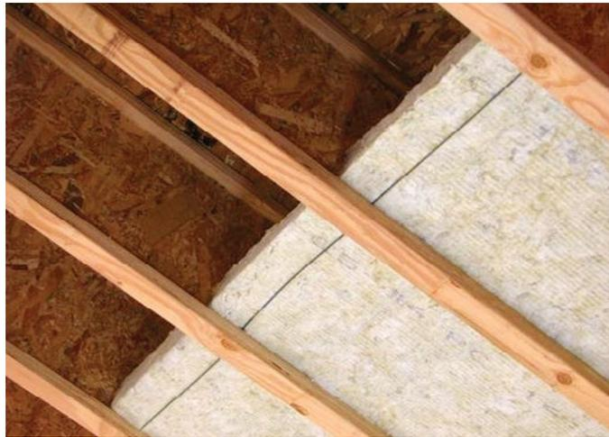
Installing mineral wool between I-joists is one of several methods builders and installers can use to meet the IRC provisions.
